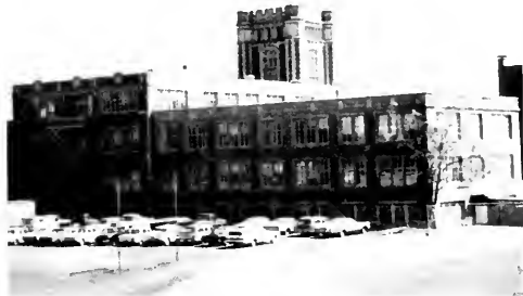
Photo 1. Los Angeles High School. Parapet and veneer shaken off four-story portion of this pre-Field Act school building.
